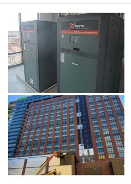
As it is the XTherm Water Heater Boilers are great for high volume domestic water heating. Plumbers love them as all components on the 2 million BTU and lower are included in the equipment which means not having to pipe external to the unit and is a huge labor saver. We like them due to the simplicity of start-up, programming, and controls.
