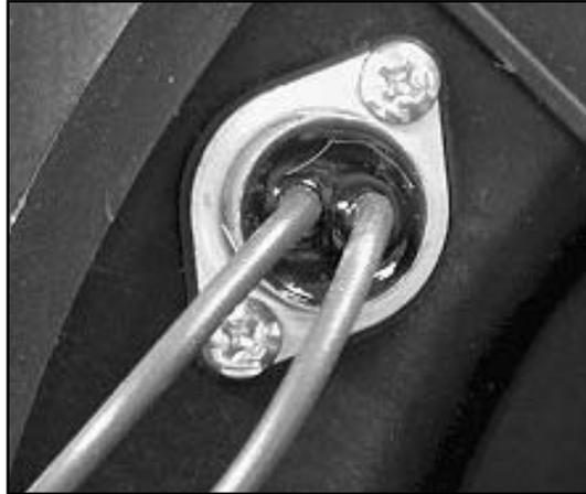
Figure 6 - Vent Over Temperature Safety Switch
