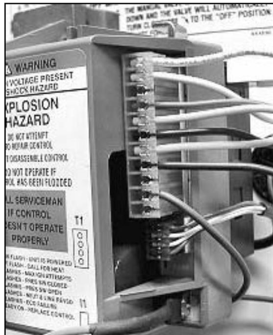
Figure 5 - 2000 Wiper Gas Control
