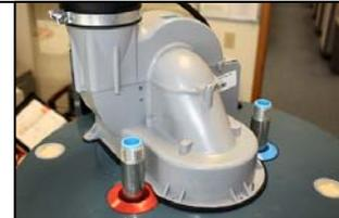
7. Remove the plastic cap to expose the anode rod.
