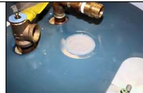
8. If not clearly visible down to the tank shell, take a flat blade screwdriver and carefully remove the insulation and expose the anode rod head.
